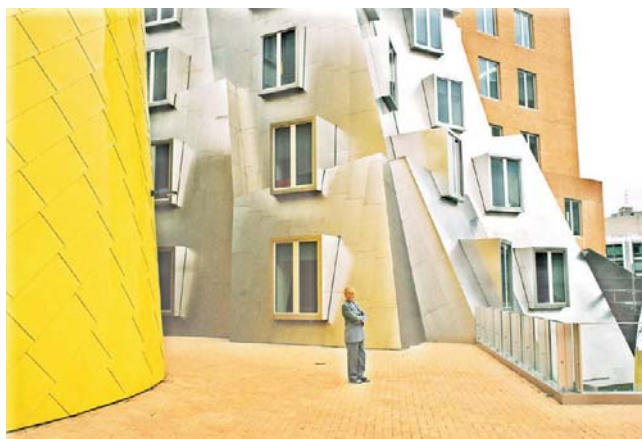
Plate 16. Stata Centre, Massachusetts Institute of Technology, Boston.
