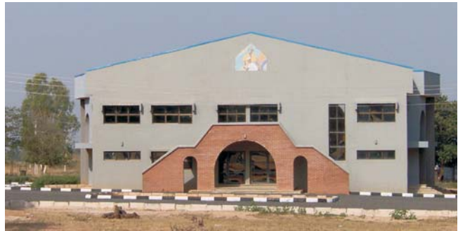
Plate 34. Multipurpose Hall, Federal University of Technology, Yola.
