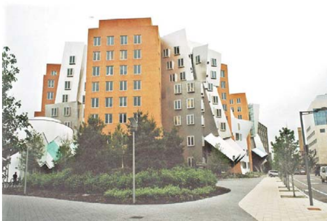
Plate 5. Stata Centre. Massachusetts Institute of Technology, Boston.
