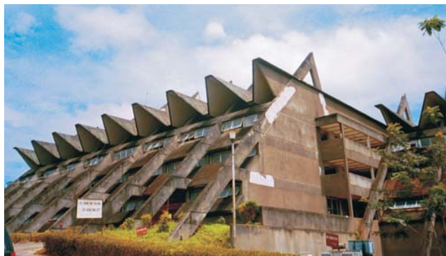
Plate 24. Civil Engineering Complex (Spider Building), Obafemi Awolowo University, Ile Ife.
