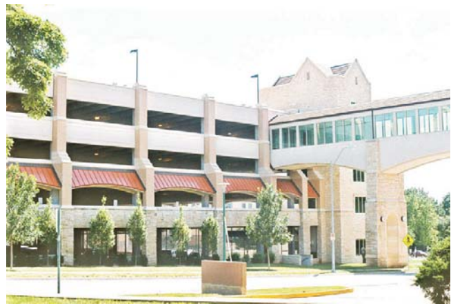
Plate 20. Multi-storey car park with bridge at the University of Missouri, Kansas City.
